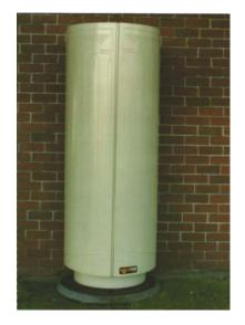
Air source system with passive evaporator wrapped around the tank.
