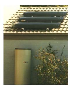
Solar boosted system with evaporator on the roof.
