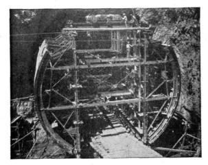
Such activities as pouring three-foot concrete circular walls by means of this fifty-foot mold which travels on tracks, are all in the day's work at Hoover Dam site. See this spectacular engineering project in the making, enroute to or from Southern California via Union Pacific's Overland Route.
